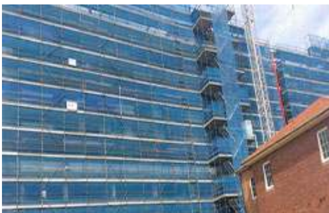
Liverpool, NSW 30 units+shops
